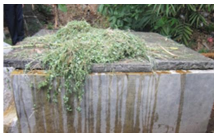
Gambar 7 Bak Residu (Sludge)
