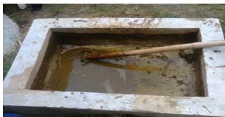
Gambar 5 Bak inlet (slurry)
